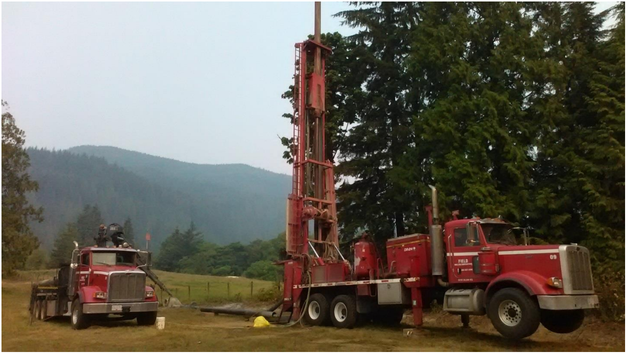
Photo 3: Truck-mounted Foremost DR-24 dual mode air rotary well drilling rig set up on PW17-1.
