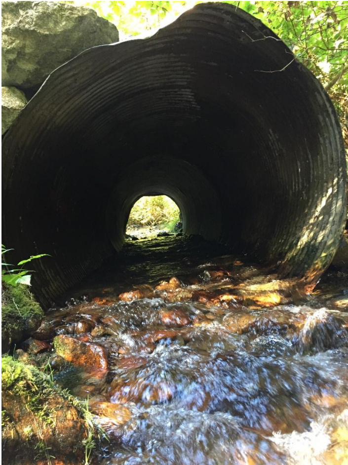
Photo 2: Discharge monitoring station on Durieu Creek.
