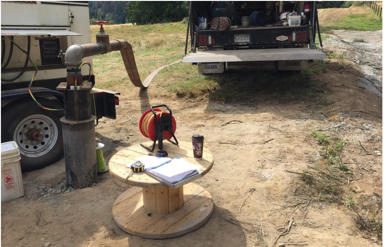
Photo 4: PW17-1 wellhead with test pump in place.
